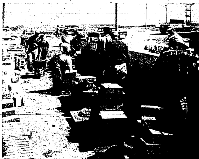
Bricklayers from Magic Valley communities work on west wall of first permanent brick building at the Idaho Ranch for Youth near Rupert. In the first day of work, walls of the structure were turned to window-all level. Some 18 bricklayers and electricians fanned out Saturday. Other work days are planned on successive Saturdays until the building is complete. (Staff photo-engraving)
