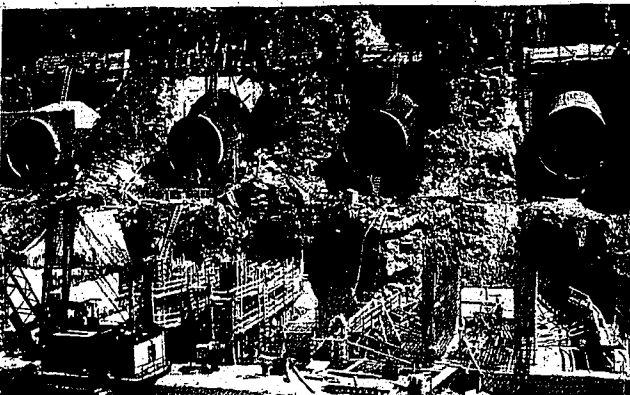
Towering mouths of four steel penstocks loom overhead as the $20,000,000 powerhouse of Idaho Power company's Oxbow dam begins to rise from the bedrock excavation at base of sheer cliff. First concrete for this mammoth structure was poured in mid-March and already it is taking recognizable shape amid a maze of timber formwork and webs of stout reinforcing steel. When completed to house Oxbow's four initial generating units, the powerhouse will be 225 feet long and 83 feet high. The penstocks will feed water to the four initial generating units from two 1,000-foot-long intake tunnels, each 35 feet in finished diameter. The tunnels will carry water from the reservoir on one side to the penstocks on the opposite side. (Staff engraving)
