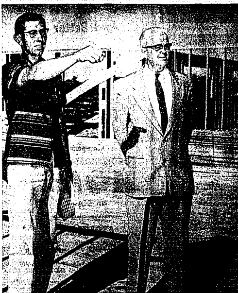
Don Oltman and Dr. Ralph A. Drake, left and right, co-partners of the new Sky View Manor, nursing home for the aged, view progress of construction on the $100,000 building. Construction began May 1, and is expected to be completed the latter part of September or first of October. There will be 72 beds, featured with a large picture window in each room. The building is located on the corner of Wendell and Fifth avenues, just north of Magic Valley Memorial hospital. (Staff photo-encraving)
