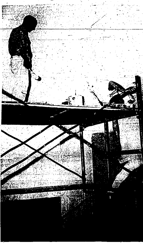
Renovation is one of many jobs that keep school teachers busy during the so-called "vacation" months. Painting a wall in Washington school auditorium are Jerry Kleinkopf, high school physical education teacher, left, and stretching an out-of-the-way spot is Clarence Parker, junior high school mathematics teacher. (Staff photo.)
