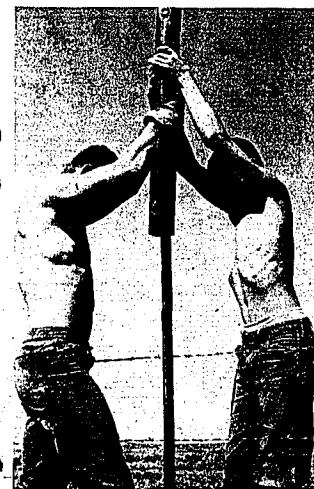
Mare Hastings, left, and Dick Greenfield hoist on the 25-pound fence post driver and drive another post in the three miles of fencing they, and other boys on the ranch, have constructed since school was out. (Staff photo-engraving)
