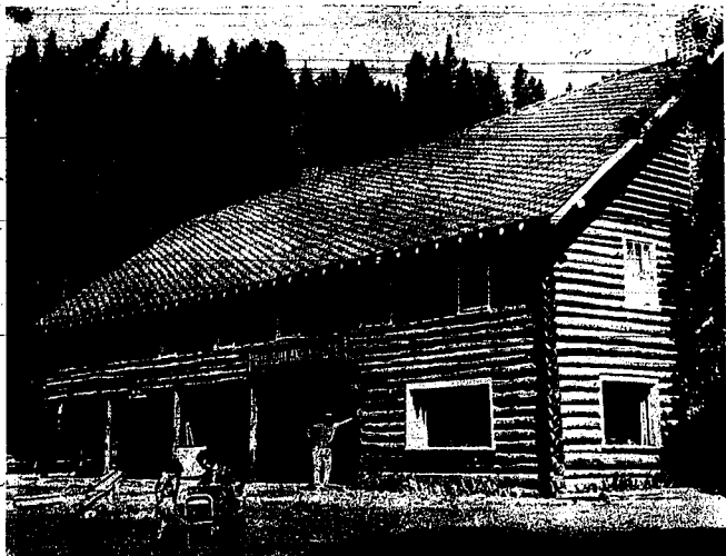
Thomas LaMore stands on the front porch of the newly redecorated Swedish Lake lodge. The area between the LaMores' stands and the nearest corner of the building has been partitioned off and converted into the new lounge. The dining room area, behind La-
