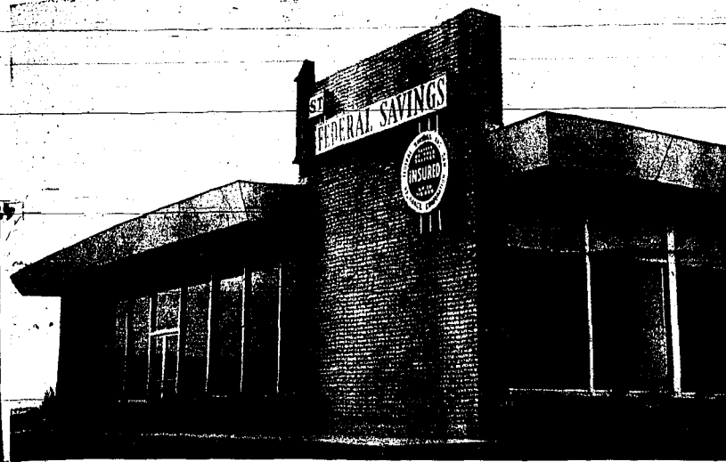
Above is the new Burley branch of the First Federal Savings and Loan association of Twin Falls which will hold a grand opening Saturday from 11 a.m. to 9 p.m. The building is located in the Overland Shopping center. It was built by Jensen Construction Co.
