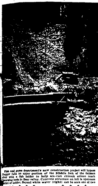
Fish and game department's new construction project will bypass Dagger Falls on upper portion of the Middle fork of the Salmon river with a fish ladder to help sea-run chinook salmon reach spawning beds in Bear Valley. Concrete structure on left is upstream end of ladder. Beyond white water (right) can be seen one of two...
