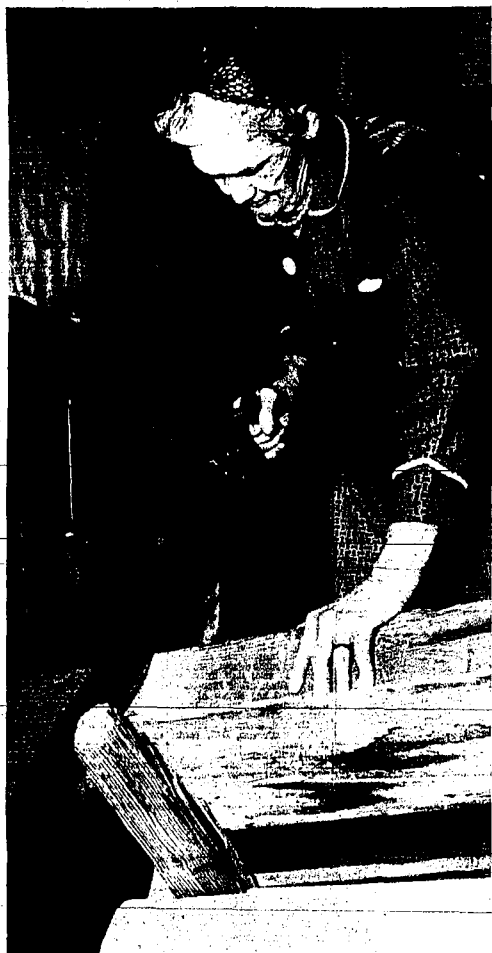
Mrs. Mary Eggleston Florj, 52-year-old part-time carpenter, sets to work with her saw. She is finishing a remodeling job on her back porch first house. Mrs. Florj says the work is tiring, but she says she couldn't get a carpenter to undertake the small job so she decided to do it herself. (Staff photo—engraving)
