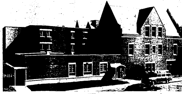
The new $390,000 addition to the University of Idaho state hospital, financed by student fees, has more than doubled the capacity of the original clinic and hospital built in 1927 when enrollment was lower. (University press service—staff photographing)
