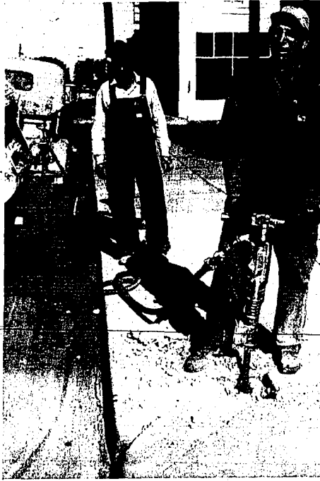
Arla Baughman, employee of the Twin Falls city street department, punches another hole for relocation of a parking meter as he prepares, Henry Selick, stands by to remove the broken counter. The men are changing the meters on Second avenue west for the proposed one-way traffic system. (Staff photo-courtesy)
