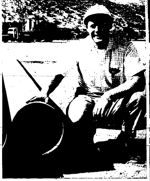
Eugene Burdick, Jerome, resident engineer for the Idaho department of highways and state engineer in charge of the new bridge across Snake river on highway 30, points to one of the 40-foot, 34-inch steel pilings used in the bridge construction. To get them in the place where they were driven in the river bed, they were plugged and floated on the surface of the water. (Staff photo-entouring)
