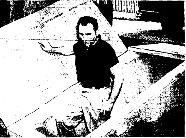
William Haffner emerges from the bomb shelter he built in his back yard just a period of six weeks spare time activity. The entrance opens into an underground chamber containing 4075 cubic feet of living space. The room is stocked with enough provisions to supply the basic needs of five persons for two weeks. (Staff photo-engraving)
