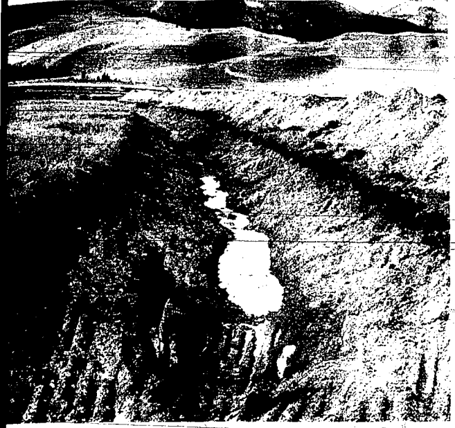
Deep ditches are being dug across the Vat creek meadow to drain away excess water... The forest service hopes to drain 400 acres of the meadow that has always been too wet to be used as grazing land.
