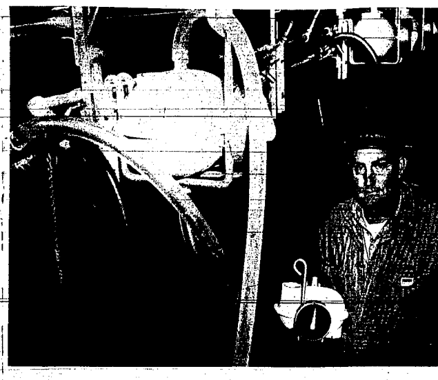
The views are shown of the milk meter, a measuring device used in dairy barns that has been introduced only recently in Magic Valley. Richard Dohse, Kimberley dairyman who has been expanding his barn and recently has purchased a bulk tank, is holding the meter so that the dial can be seen. The other meter, in white and to the front left, is in place in the pipeline with hoses attached. The
