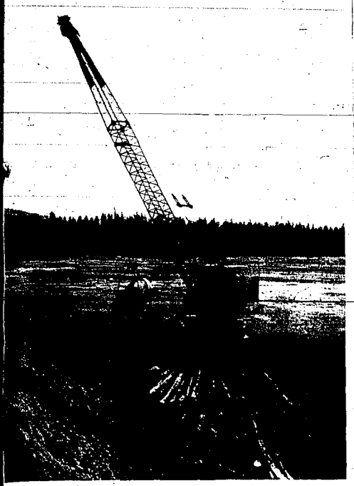
This large dragline is working currently on a swamp draining project on Vat creek in Sawtooth valley. The forest service is experimenting with the drainage project and hopes to drain the area by lowering the water table and add about 400 more grazing acres to the Vat creek meadow. (Staff photo-entourage)
