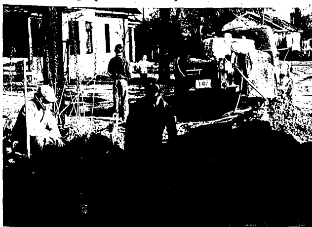
Paul's Cuffman, left, and Carl Crook, repair a break in a 30-inch water main at the intersection of the after between Second and Third avenues north and 23rd street north. The main started leaking Thursday evening and a section of the main broke about midnight while men from the water department were attempting to repair the leak. (Staff photo-enlarging)
