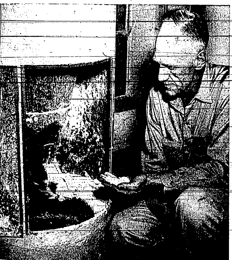
Earl Fuller, plant operator, holds some of the powdered alum in his hand at the bottom of the large alum hopper. It is here that the alum is fed slowly into the water, which circulates through the base of the hopper. (Staff photo-engraving)
