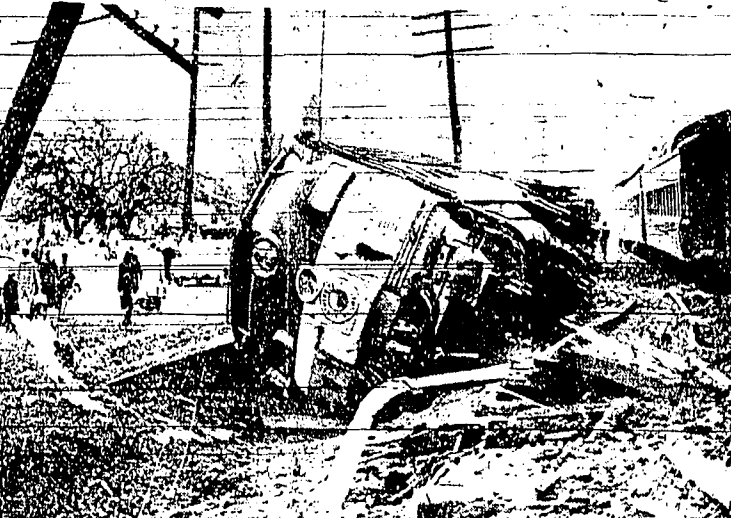
This is the diesel engine pulling a 17-car Northern Pacific passenger train, after it plunged off tracks, overturned and plowed into a ground at Puyallup, Wash. Officials said it was caused by a broken rail. (AP wire photo)
