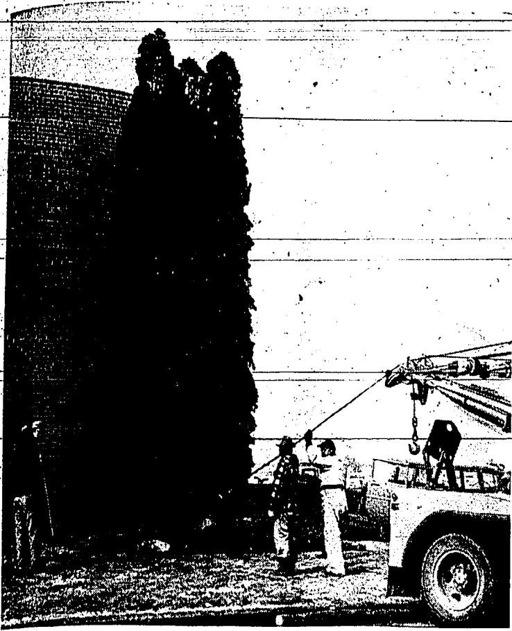
Members of the Twin Falls Grange led by T. (Pete) Creed, second from right, are shown placing two large 45-year-old pines on the east side of Maglo Valley Memorial hospital Tuesday. They were assisted by Doyle and Keith Sligar, operators of the Thousand Springs resort at Hagerman. The Sligars donated the services of the truck. The trees were donated by Herschel Sonner, 102-year-old Maglo Valley resident. (Staff photo-engraving)
