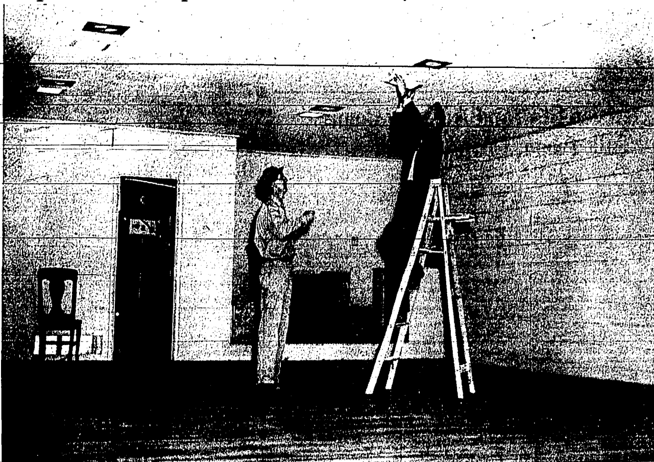
Andrew (Andy) Baird, left, and William Coffield put the finishing touches on a new square dance hall in Twin Falls. Baird is president of the Southcentral Idaho Square Dancing association and the building is located on Blue Lakes boulevard north. Several local square dancing clubs will use the hall. The hall is well-lighted and has 10 loudspeakers mounted in the ceiling to carry the caller's voice to the dancers. (Staff photo-engraving)
