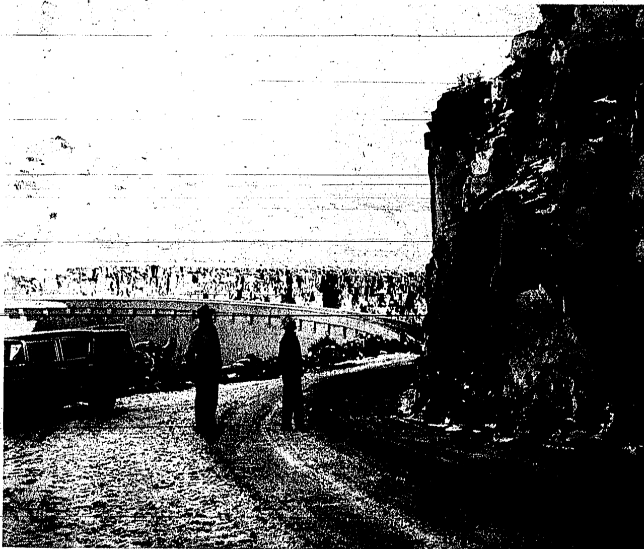
Floyd Dayley, left, assistant director of the Twin Falls highway district, and W. E. Chase, chairman of the board of directors, look over the improved grade on the west side of Salmon dam. Until recently, the grade has been a one-way road, drawn to one-way traffic only on the road across the dam. The road was about 12 feet wide, now it is 22 feet wide and a turn-out area (where the car is parked) has been constructed about half way up the grade. Much rock was blasted from the side of the hill in courses of many drivers over the years. Now the road is a two-way road, harrowing to widen the road. (Staff photo-engraving)
