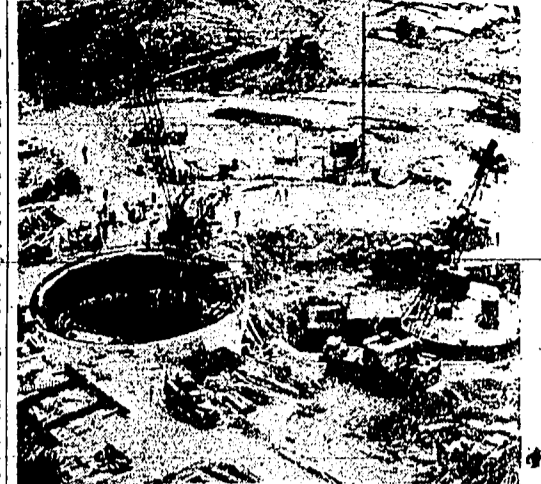
The Atlas missile site silo at Roswell, N. M., where six men were killed Thursday is seen in this aerial view. The silo is 170 feet deep and 40 or more feet in diameter. The men died when a crane similar to the one being used to lift the wrecked crane from the hole tumbled into the excavation and exploded. Fourteen other men were injured. (AP wirephoto)
