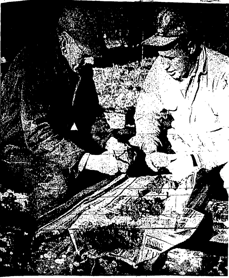
Bill Martin, right, well driller, discusses with Mervyn Esterhold the importance of sand and gravel samplings. According to Martin, sand and gravel are good indications of a good water supply. Those seen were obtained from 30 feet below ground level. Martin expects the well to be dug to a depth of 100 to 150 feet, and will be completed the end of the week. (Staff photo-engraving)
