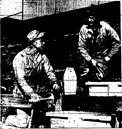
Clyde Biggers, left, park attendant, and Howard Johnson, maintenance superintendent, work at replacing the Jaycee park bleachers. In the past few weeks thousands of board feet of lumber have been used to make spot repairs on the bleachers. A new set of rest rooms has been installed and, when the weather warms, the bleachers will be repainted. (Staff photo-engraving)
