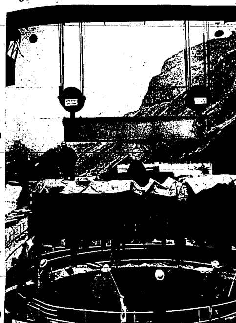
Down into position goes 220-ton rotor for first of four generators that will start spinning out electricity this year at Idaho Power company's 220,000-kilowatt Osbow dam. About 27 feet in diameter, rotor is seen covered with paper as protection against heavy rain that was falling at permanent purchase pany crane carefully lowered it into place. Workmen stationed around unit help guide rotor into position. Gomer Condit, Idaho Power resident engineer, said rotor was one of last of many massive pieces of equipment to be installed for first generator. Rotor, connected by shaft to turbine, will turn within so-called "starter" to produce electricity. With rotor turning at 94.7 revolutions per minute, its outer edge will be traveling at more than 90 miles per hour. (Idaho Power company photo-staff engraving)
