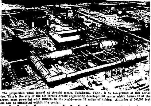
The propulsion wind tunnel at Arnold center, Tullahoma, Tenn., is in foreground of this view. This is the site of the air force's Arnold engineering development center which houses 12 of the largest, most powerful wind tunnels in the world—some 16 miles of tubing. Altitudes of 200,000 feet also can be simulated within the center.
