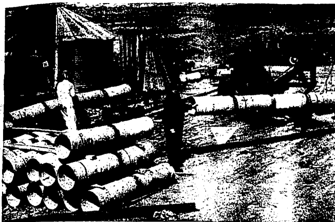
This is a scene at the busy factory outside of Hagerman that is putting the four-foot incendiary bomb casings together into 60-foot lengths. They are then hauled to the construction site southeast of Hagerman. Emerson Pugmire, center, estimates that the
