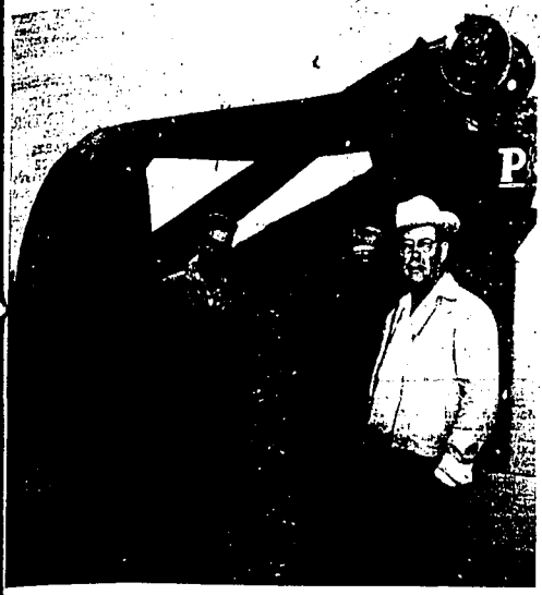
Because the Salmon River Canal company, Hollister, purchased a Back-hoe for this crane about a month ago, it was able to install a pipeline in a company lateral that will save an astonishing amount of water in one area during this season. The area involves only three farms, but the pipeline will save about 1.5 acre-feet of water on a 21-hour run. In money, the value of this water will exceed $2,000 for the season. From left are Leslie Jones and Lyle Schmitzer, canal company board members, and H. M. (Pete) Griffith, canal company manager. (Staff photo-rewriting)
