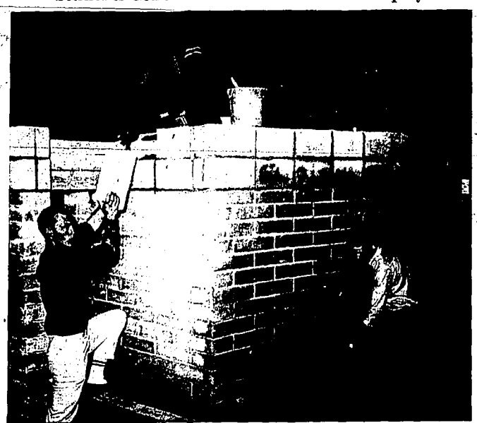
Students put the finishing touches on a fallout shelter in the Twin Falls high school shop building. On April 30 the shelter will be on display to the public. Students who worked on the project are, from left, Dale Willis, son of Mr. and Mrs. Earl Willis; Don McDowell, son of Mr. and Mrs. Sidney McDowell; and Harold McCollum, son of Mr. and Mrs. Paul McCollum. (Staff photo-engraving)
