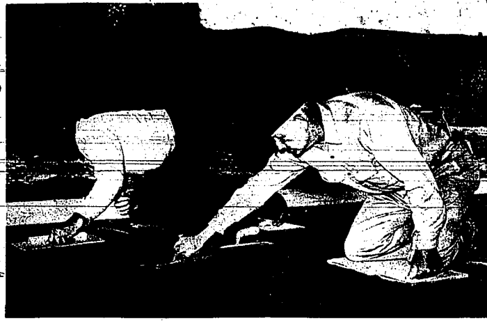
Two volunteer workers put the finishing touches on the floor of the new shelter house at Niagara springs. They are Elmer Young, left, Orchard Valley, and Mrs. Kistler, Gooding. The volunteer workers from the Magic Valley area recently have completed two new projects at the recreational area—a shelter house and a concrete slab for dancing or shuffleboard. The labor for the new shelter was donated by members of the Gooding Pomona Grange and its seven subordinate Granges. (Staff photo-graving.)
