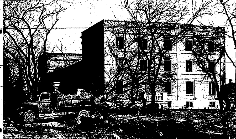
The Park hotel once was a landmark in Twin Falls but can be remembered now only in photographs. The hotel, once a hospital, is being razed to make way for the new Twin Falls postoffice. The hotel was first built as a hospital in 1906. It was called the Boyd hospital. Later it was converted into a hotel, and operated as such until recently. For many years it was one of the finest hotels in southern Idaho and was the site of many convocations and was the meeting place of most of the town's clubs. The hotel grounds were also the site where a body of a murdered man was found and sparked one of Idaho's most sensational murders. (Staff photo-enshrining)
