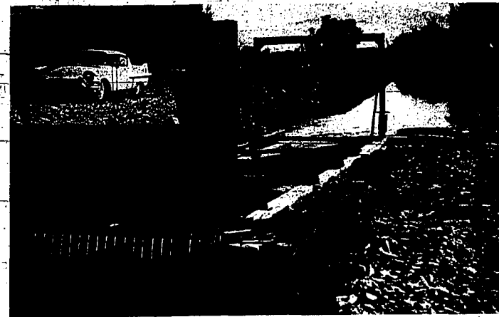
Fish and game department fish screen of the louver type has been designed, built and installed on experimental base near Salmon City. It consists of a vertical "venetian blind" stretched across ditch entrance. Water passes through but bypass fish away from the obstruction and are drawn into a bypass flow.
