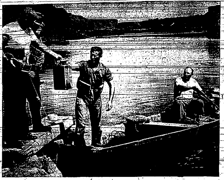
Workers get ready to leave the bank of Snake river to blast rocks out of the middle of the river. Using 1,000 pounds of dynamite, they blasted a channel through the rocky area above the Niagara Springs recreational area, adding about 10 more miles of navigable water. Boaters now can ride all the way to Auger Falls above the confluence of Snake river and Rock creek. From left are Buck Cherry, Emerson Pugmire, Gene Padgett and Mac Dugan, all Hagerman. (Staff photo- engraving)
