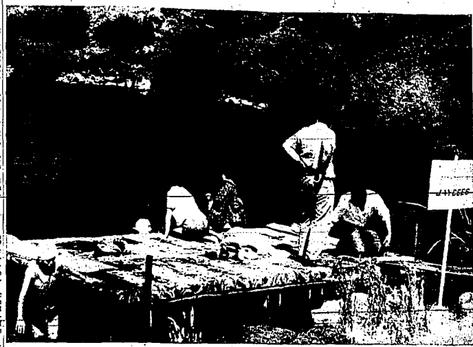
Dick Messersmith, swinging hammer, and Leroy Dodson, chairman of the Twin Falls Junior Chamber of Commerce boat dock project at Shoshone Falls, work on the ramp as sunbathers make use of the completed portion of the 12-foot dock.
