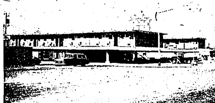
Each of the 30 units in Boise's new and modern "Sun-Liner" motel, located on Highway 20 in Garden City, has its own individual electric heat pump to provide summer cooling as well as winter heating. *TM REG US PAT OFF
