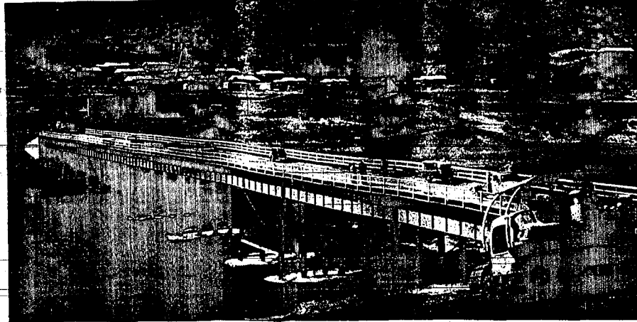
Some 500 feet long from shore to shore, this is modern two-lane bridge across the Snake river that workmen have completed as the first major step in construction of Idaho Power company's Hells Canyon dam project. Use of new span, located just below Otbow dam, will be limited temporarily to men and heavy equipment engaged in pushing a 23-mile access road downstream along the Idaho side of the river to the Hells canyon site. Later it will be opened to the public as the "hub" of a network of new roads providing faster, safer access to the Hells canyon and Seven Devils country. (Staff engraving)
