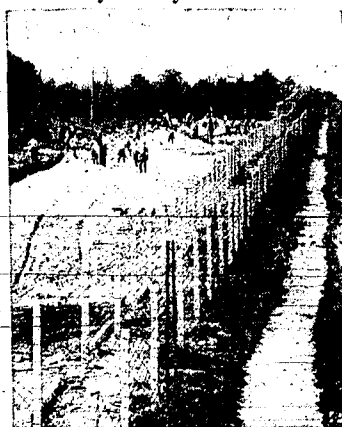
Workers level rubble of houses demolished behind wire fences, on east side of Berlin to eliminate one means of escape by East Germans. (AP wirephoto)
