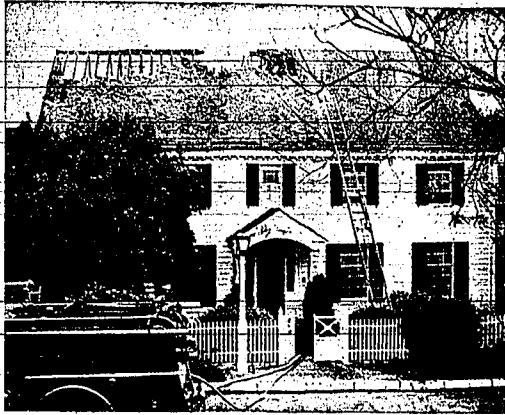
Part of the roof is gone from the home of actor Fred MacMurray in the suburban Brentwood area of Los Angeles as result of the disastrous brush fire. The upper floor also was damaged. MacMurray rushed home from his television film set to help move his family and their belongings. Mrs. MacMurray, actress June Haver, and their 5-year-old twins were not injured. (AP wirephoto)
