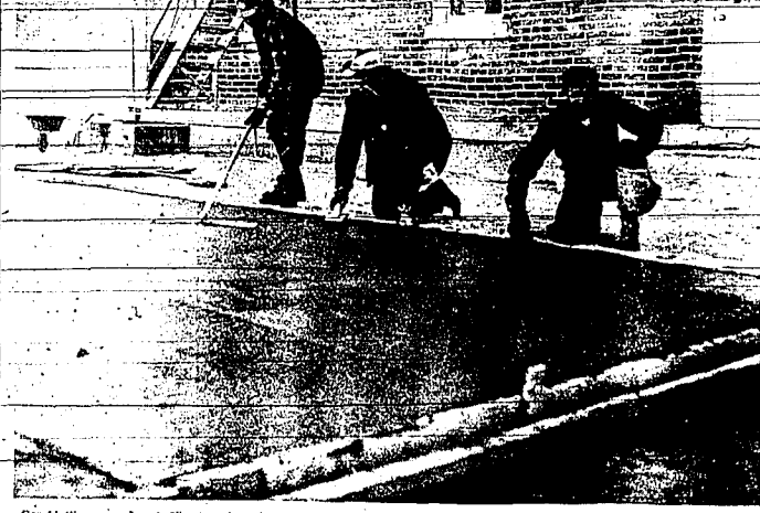
Gerald Sherman, Joseph Wurst and Ed Peck, from left, put finishing touches on a 50-by-35-foot slab of concrete poured at the rear of the Bellevue school, Lester Lewis, school principal, says the space will eliminate mud brought tracked into building. The work was done by volunteers from the Bellevue P.T.A. (Staff photo-gramming)
