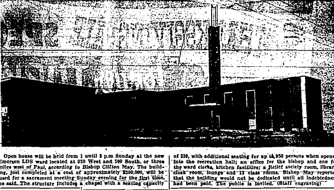
Open house will be held from 1 until 5 p.m. Sunday at the new Emerson LDS ward located at 350 West and 100 South...
