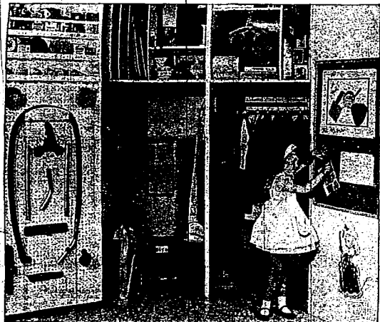
Playroom nook housing heavily insulated water heater can be turned into a bonus storage area. Perforated doors permit circulation of air.
