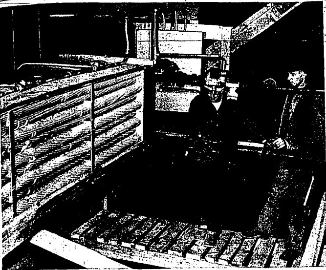
REFRIGERATION SYSTEM gets a last-minute inspection by two workers high on a catwalk near the ceiling of the warehouse. They are Lee Edwards, left, electrician crew foreman, and Mel Howell, refrigeration supervisor. The big refrigeration system measures nearly 80 tons. The new warehouse is located on highway 30 west of Burley. (Staff photo-enslaving)
