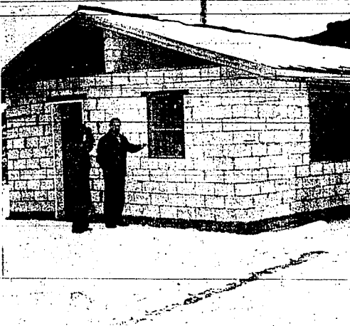
TESTING BARRED WINDOW of a 28- by 20-foot cinderblock building at Shoshone falls is Ernest Craner, right, superintendent of parks and recreation department. In the building will be two modern restrooms with modern facilities and a snack bar. The snack bar will serve lunches and also hand out literature to tourists about the Shoshone falls and Twin falls parks and other recreational places in Magic Valley and Southern Idaho. Howard Johnson, left, is foreman of the park. (Staff photo-engraving)
