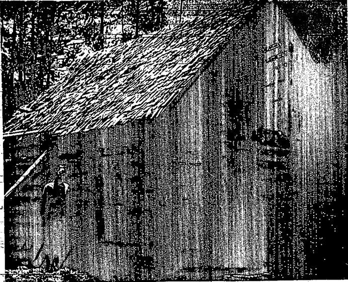
THE LAST BUILDING remaining of all those which once marked the site of Galena, first of the Wood river valley mining towns, still stands at the townsite. Constructed either in 1879, the year the town started, or in early 1880, the structure is made of heavy joined logs and roofed with shank shingles. Mrs. O. A. Kehler, Twin Falls, is shown beside the structure which will be featured at a new slide-lecture show presented by O. A. (Gus) Kehler, titled "Historic Wood River and Bayshore." (Staff engraving)
