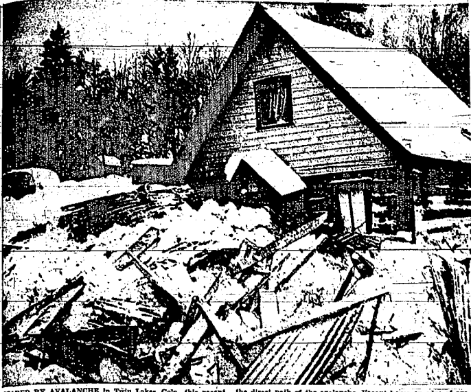
HARMED BY AVALANCHE in Twin Lakes, Colo., this vacant house on edge of woods stood next door to the house where General Shelton, his wife and three children were killed because their home was in the direct path of the avalanche. Vacant house on edge of woods had only minor damage. Debris is mixed with snow carried down mountain by avalanche. (AP wirephoto)
