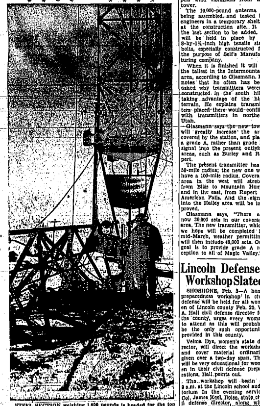
STEEL BEGINS weighing 1,000 pounds to head for the top of the tower. One of the workers' steelies is held while Kirkman operates the winch. The section will be lifted to the top and then bolted in place by three workers, who are working at a height of about 65 stories. (Staff photo-engraving)
