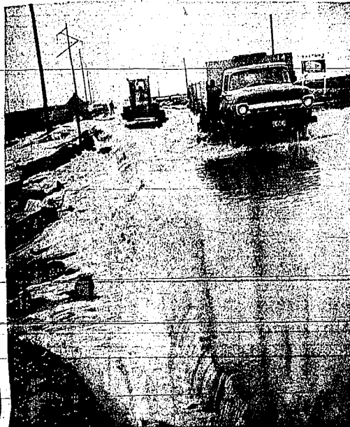
TORRENTS OF WATER flooded about 200 feet of the Meridian road, north of Rupert, and extensively damaged the road. Highway crews were busy Saturday afternoon trying to remove large chunks of ice that were blocking the shoulder of the road and blocking passage. (Staff engraving)
