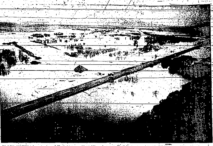
BLOOD-WATERS ran at edge of U. S. highway 88 at Mineral Springs in February as early runoff was sparked by rain and unseasonably warm temperatures. Largely as result of the early runoff, Salmon reservoir has 38,170 acre feet of water now, almost twice as much as at the same time last year. In addition, the watershed snow pack is above average. (Times-News photo)
