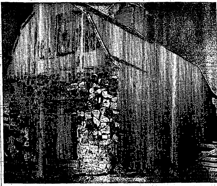
ROCK BARN is observed by Theo Gihring, owner. The barn is free for anyone who wants to come and take it. The 28- by 44-foot rock barn was built by placing rock upon rock without any sort of mortar. Mortar was added a few years ago. There is
