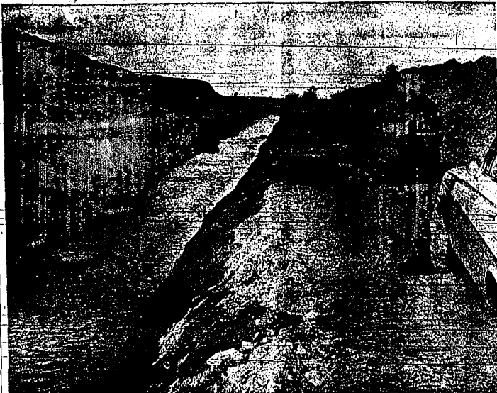
SHORTENED LATERAL is pointed out by Alfred Peters, manager of the Twin Falls Canal company. The lateral, located about five miles northwest of Buhl, was originally six miles long and now it's about four and one-half miles long, he projects.
