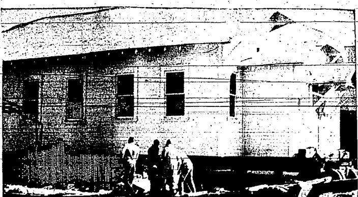
REORGANIZED LDS church building at Rupert was moved last week to a new location at Fifth street south and D street. The structure was located at Ninth and F streets since 1921 when the congregation constructed it. The lot recently was sold to the...
