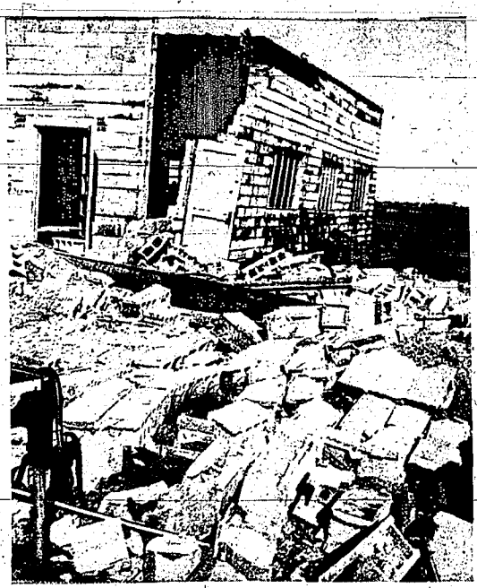
CINDERBLOCKS LITTERED area adjacent to Buritan club being built at Hickory, Va. Sunday storm scattered blocks, roof and timbers. The club was finished except for interior (left) (AP wirephoto)
