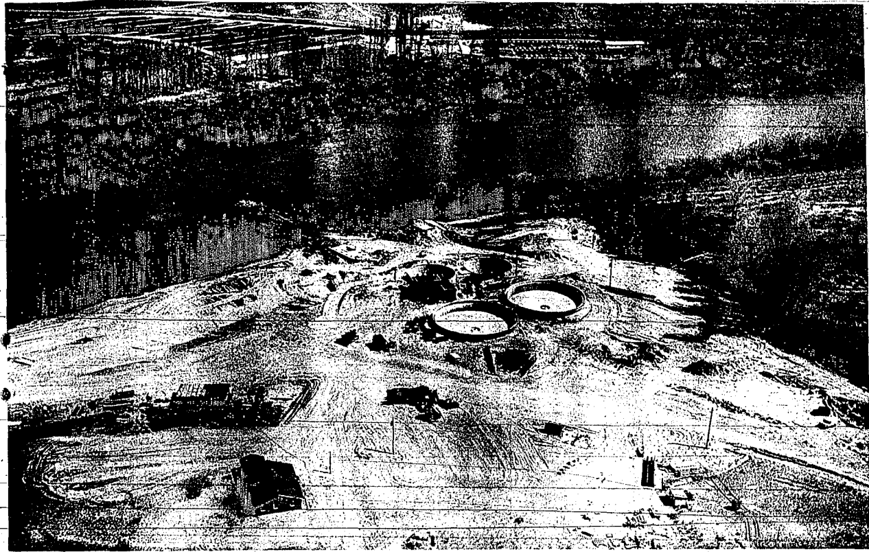
SEWAGE DISPOSAL plant for Twin Falls, now about three-fourths of the way completed, is graphically shown in this picture made from high on the south rim of Snake river canyon. The Snake river flows by the site and the Blue Lakes trout farm is visible at top of the photo. The superintendent's house is in the left foreground and the two large circular objects are the clarifiers, each 75 feet in diameter. The two smaller circular structures are digesters and are 50 feet wide. The laboratory and control house stands between the digesters and the clarifiers. Foundation of the chlorine contact chamber is seen near the river and the disposal pipe will dump into the river at the point where the dikes is seen extending. Settling basins will be constructed between the temporary work shed, left center, and the river. The entire area will be landscaped when completed. (Times-News photo)
