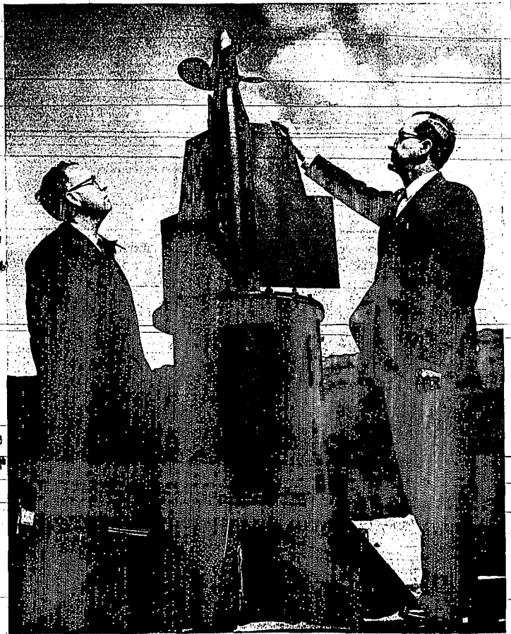
CONTROL HOUSE of the soon-to-be-completed sewage disposal plant for Twin Falls, forms the backdrop as Earl Fullmer, left, who will be plant superintendent, discusses progress with Herb Derrick, city manager. The city engineer's department reports "good progress" on the construction by Power Engineers, Inc. (Times-News photo)
